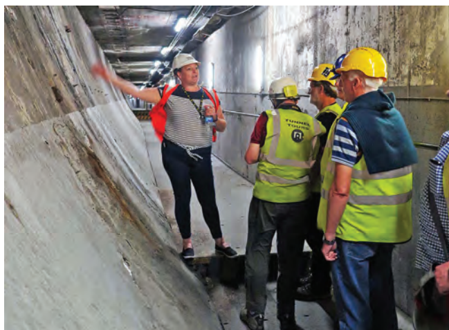
SubBritters looking at the original 1930s tunnel wall, now used to funnel clean air into the roadway. Photo Clive Penfold
